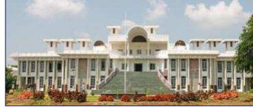
IGP Office Complex, Gulbarga Gold Rating
